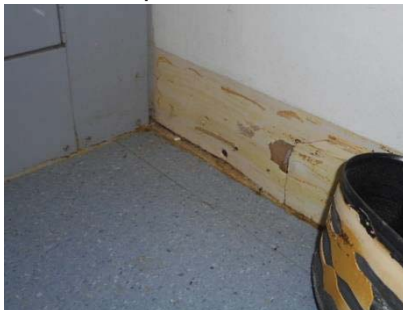
With rubber baseboard removed.
