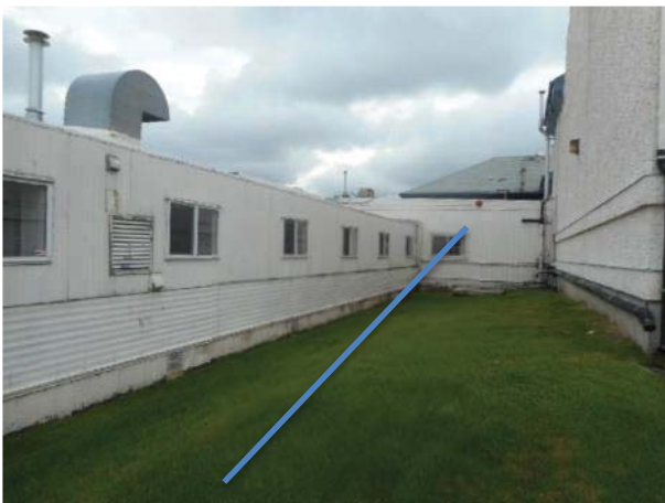
Location of FS-109 in relation to the library portable and the gymnasium. Note the gym grading towards the library and the damp shady environment created by the positioning of the portables.
