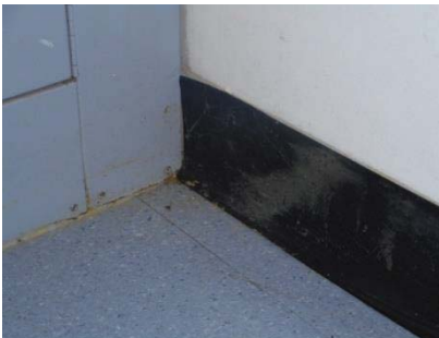
Northeast corner by furnace.
