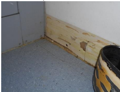
With rubber baseboard removed.
