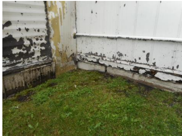
A close up of the corner where FS-109 joins the library portable.
