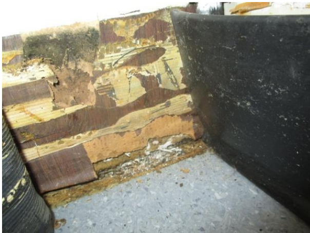
The rubber baseboard was removed from the southeast corner of the classroom.
