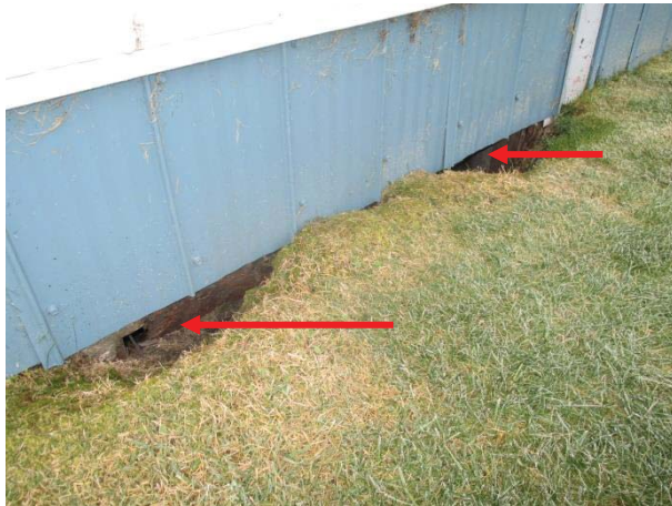
Sink holes were present along the north side of F-111 enabling water and animals to enter the crawlspace.
