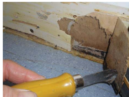
Mould growth on drywall paper Aspergillus sp. Chaetomium sp. and Stachybotrys sp.
