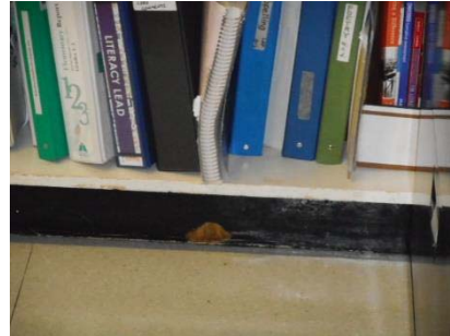
Wood rot at the bottom of the bookcase. Sample #4437.04
