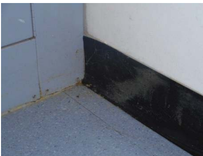
Northeast corner by furnace.
