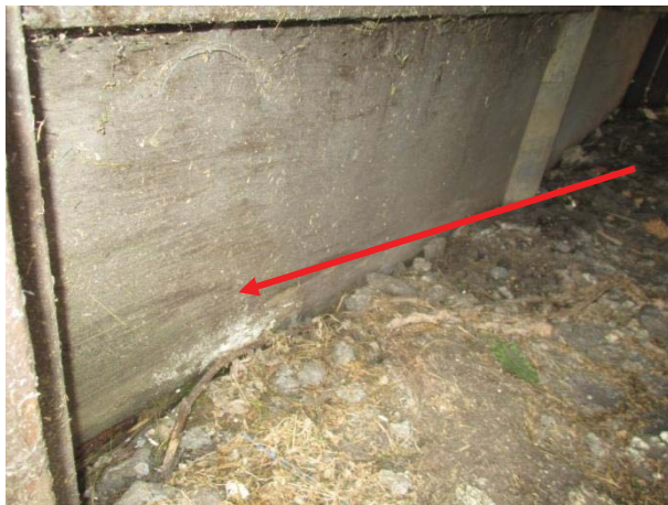
Sink holes were present along the north side of F-111 enabling water and animals to enter the crawlspace.
